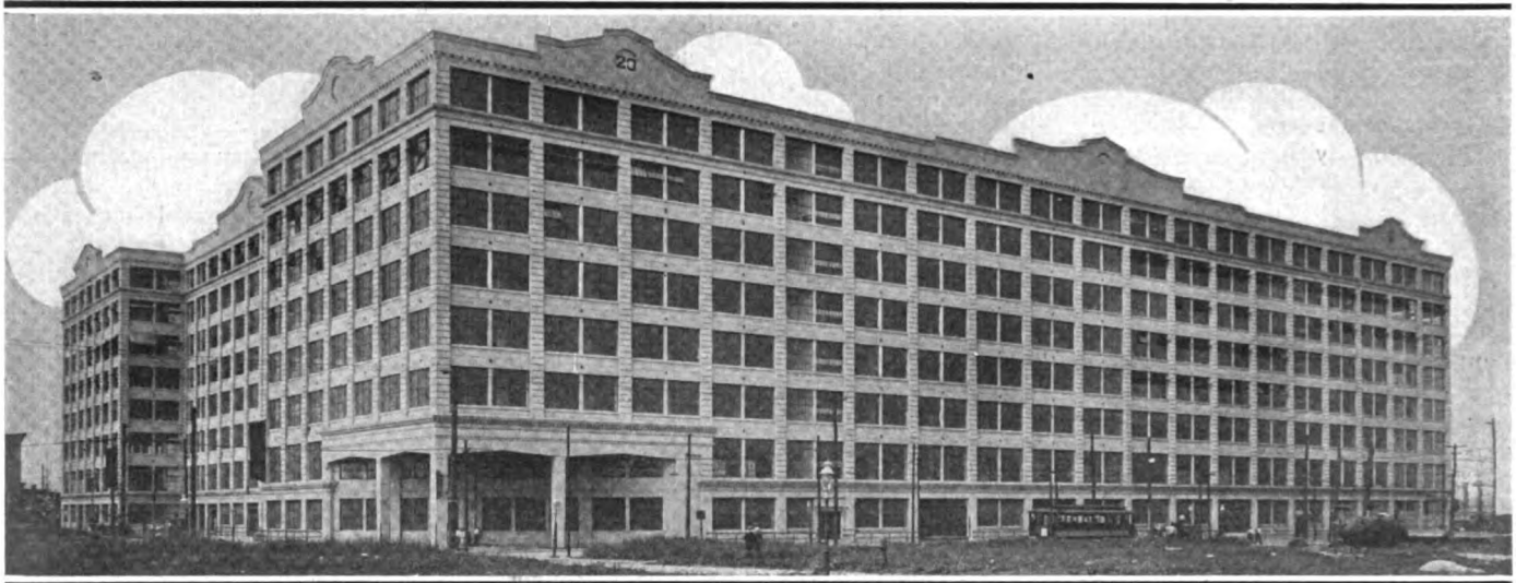
Specimen of steel reinforced concrete factory building at Bush Terminal. Tenant may have 140,000 square feet of space on one floor of this building
